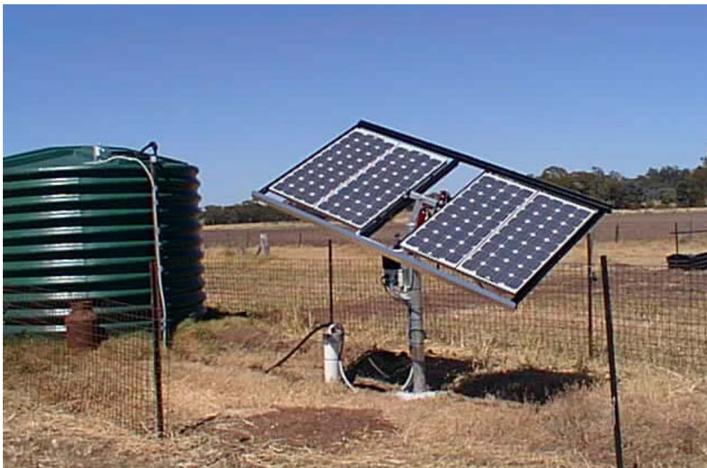
photovoltaic rack for solar pump
